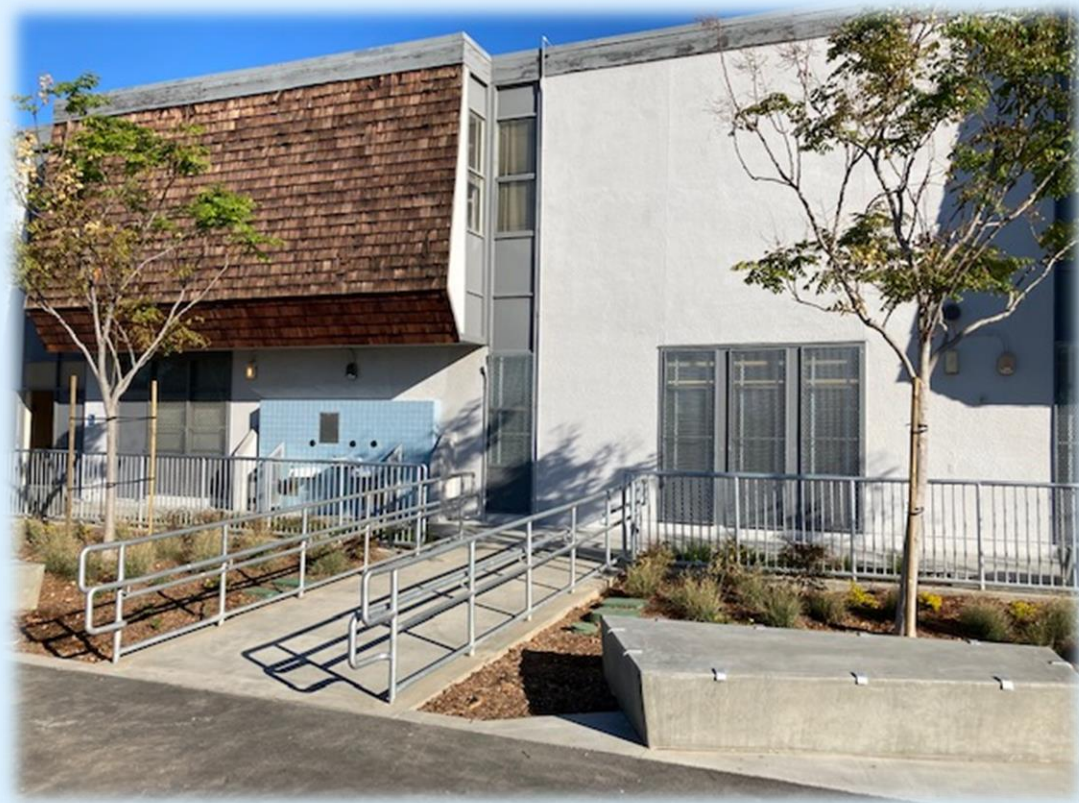
Accessible Handrail Ramp and Walkway
