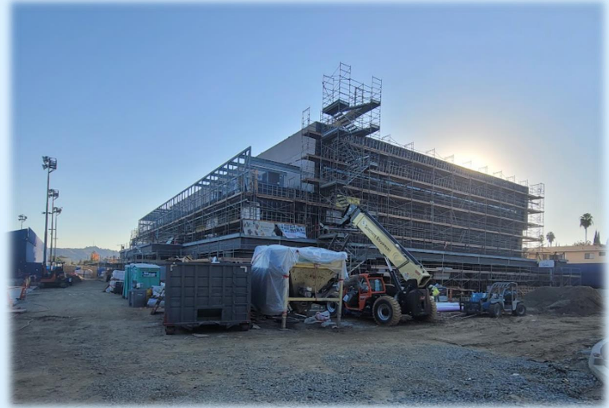
In Construction: Exterior of New Gymnasium
