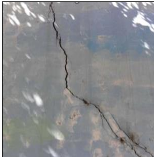
Cracked Retaining Wall
