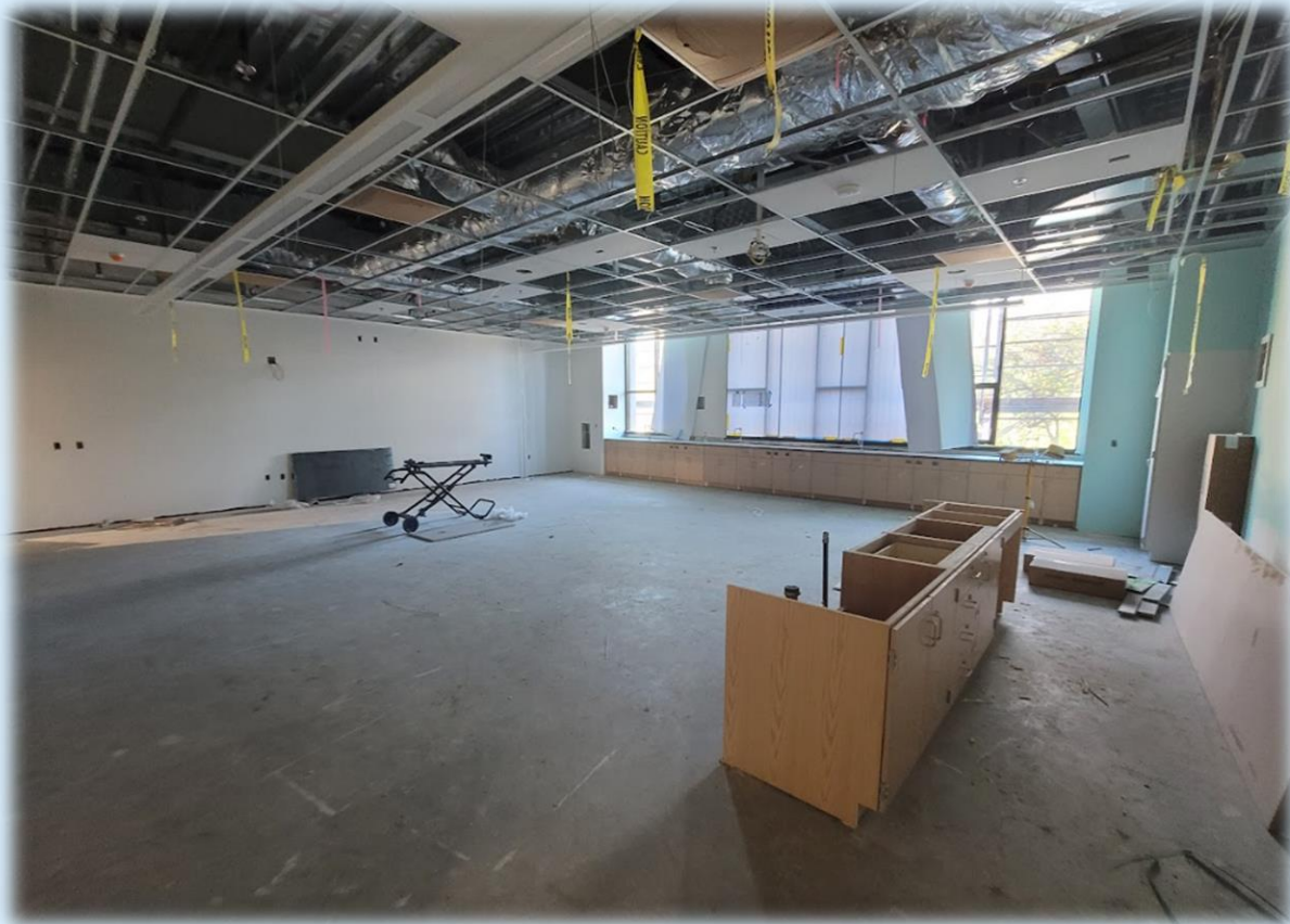
In Construction: New Science Classroom
