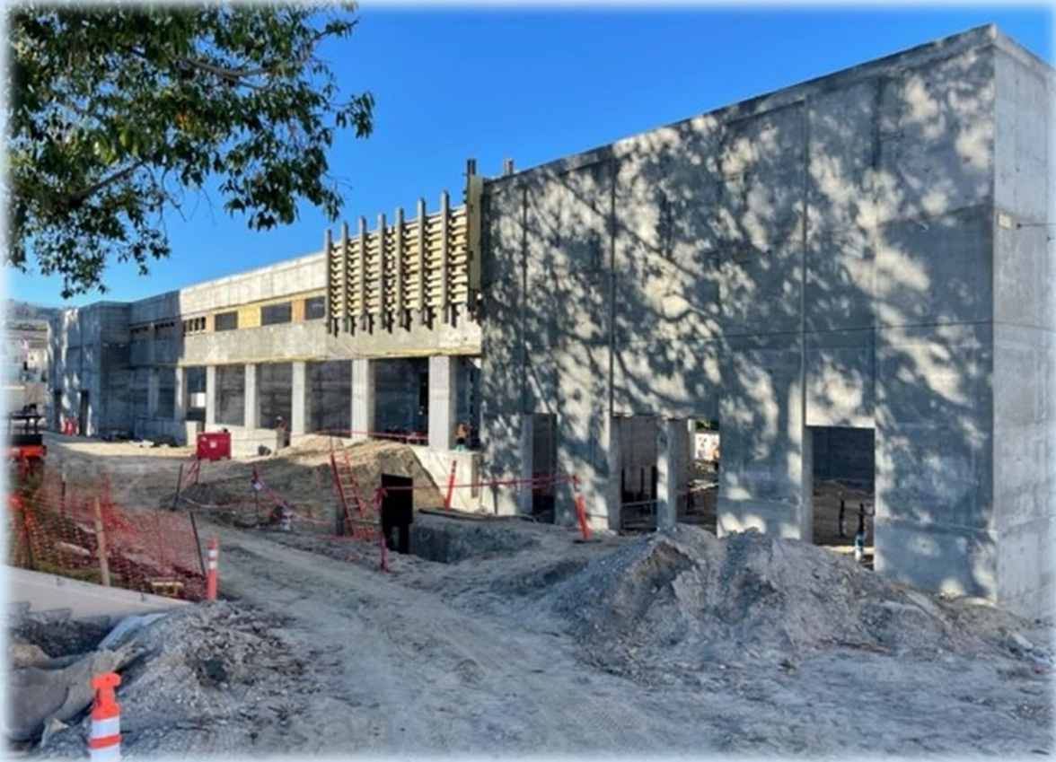
In Construction: New Visual Media/Band Building
