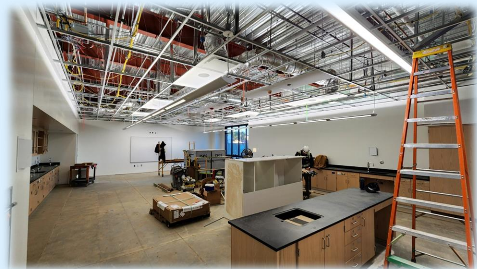
In Construction: Flex Science Room
