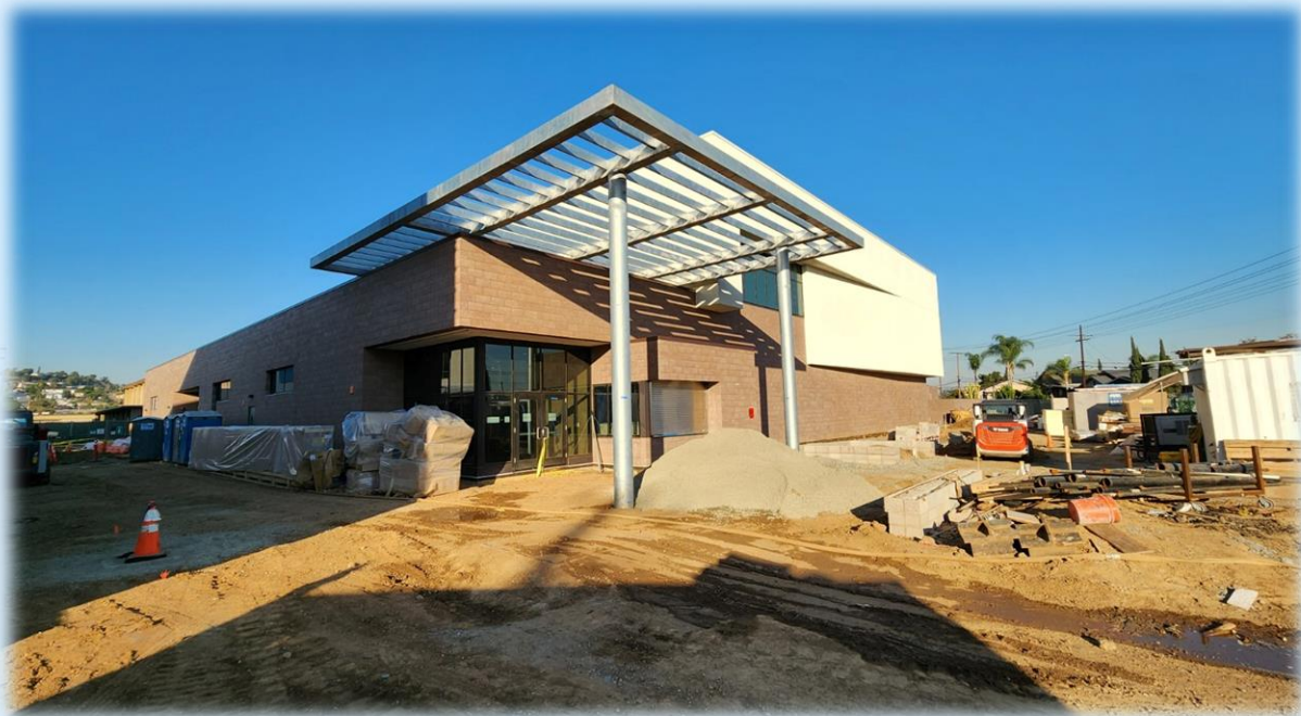
In Construction: New Gymnasium Building
