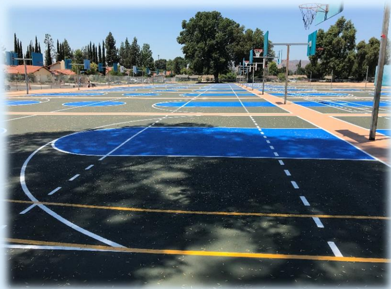
Newly Paved and Painted Play Area
