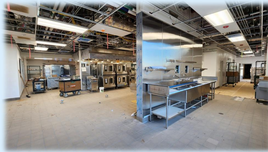
In Construction: Kitchen
