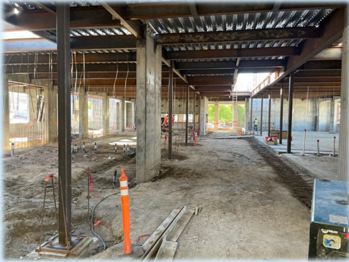
In Construction: Interior of New Administration Building
