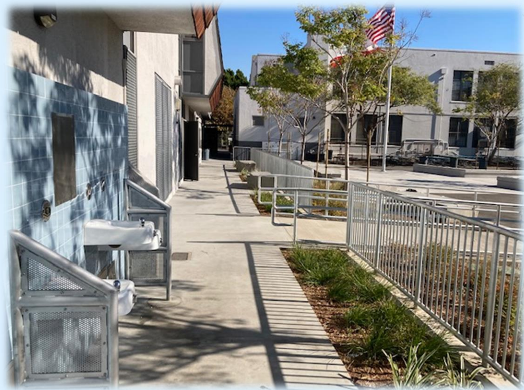
New Drinking Fountain and Walkway
