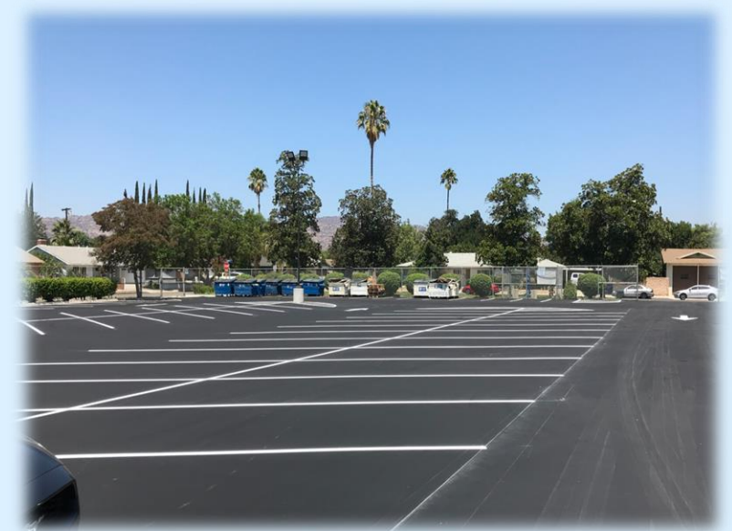
Freshly Paved Parking Lot
