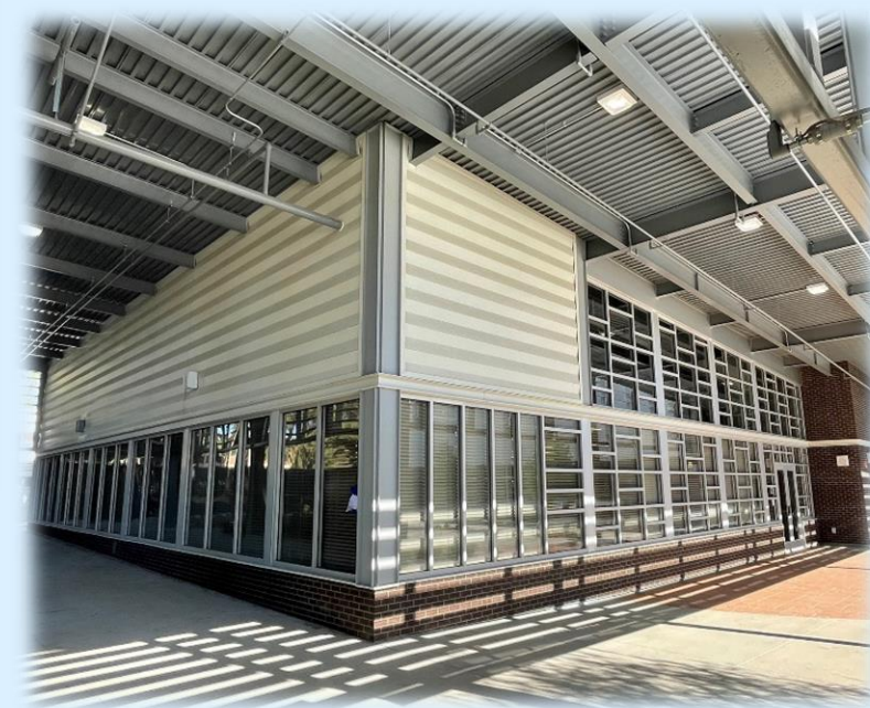
In Construction: Exterior of Library and Performing Arts Building
