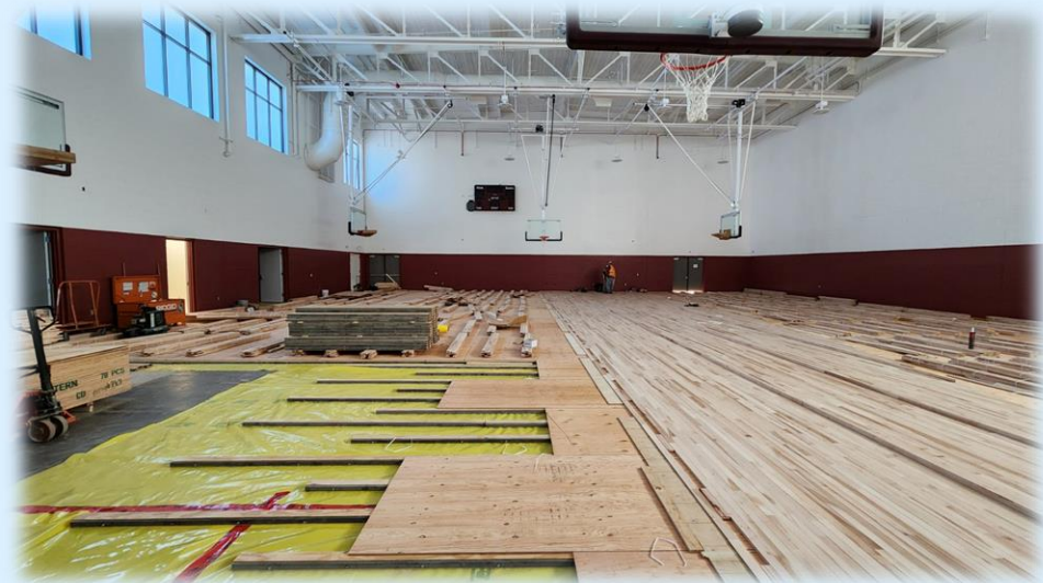
In Construction: Gymnasium
