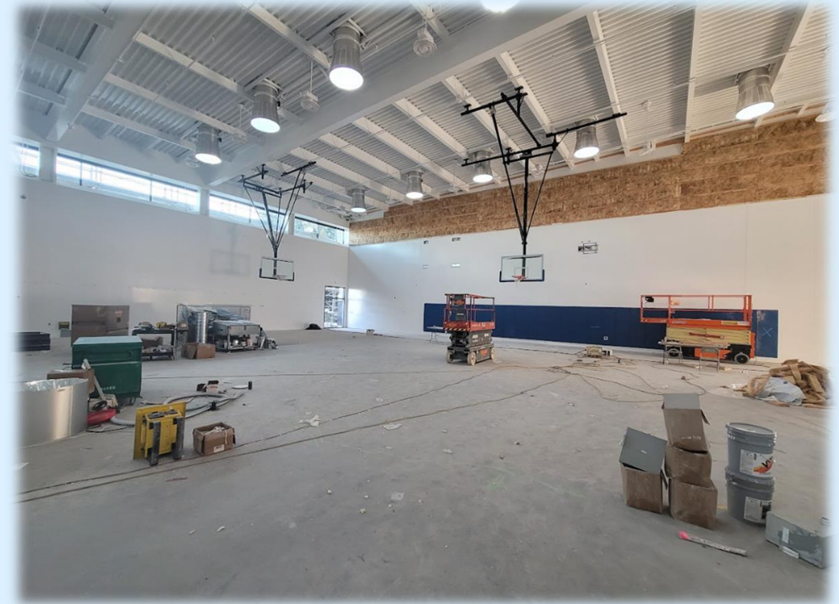
In Construction: New Gymnasium
