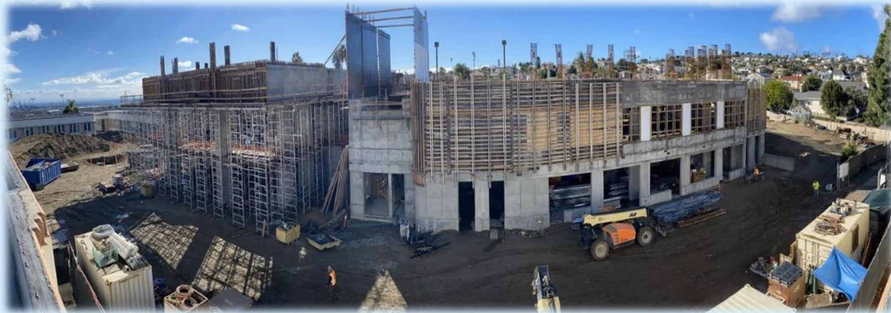
In Construction: Administration/Food Services/Classroom Building
