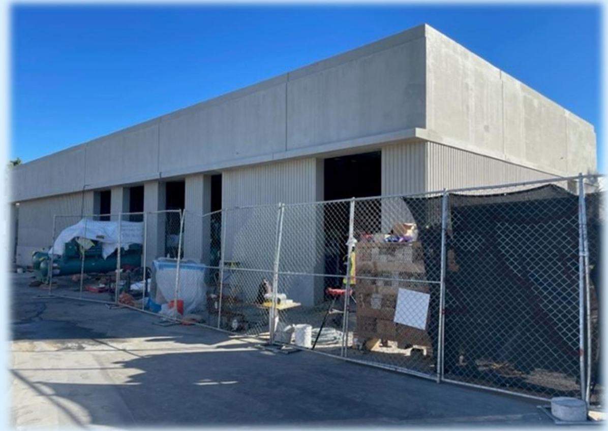
In Construction: New Central Plant Building
