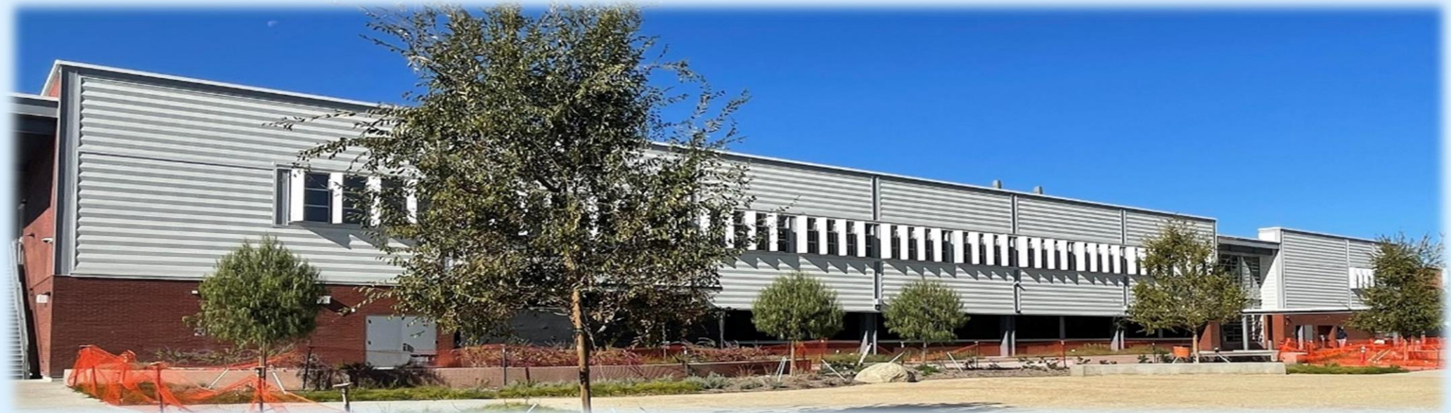
In Construction: Exterior of New Classroom Building and Courtyard
