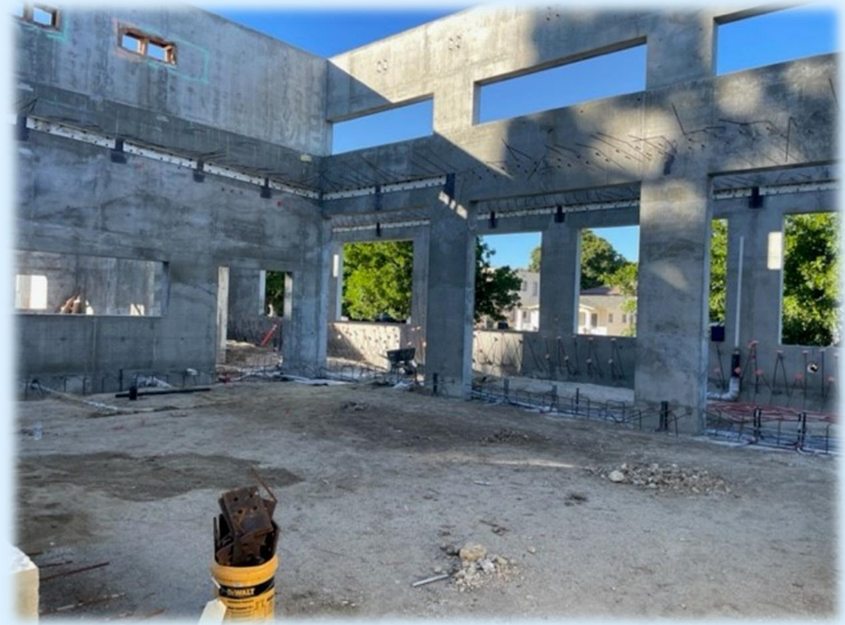
In Construction: Interior of New Visual Media/Band Building
