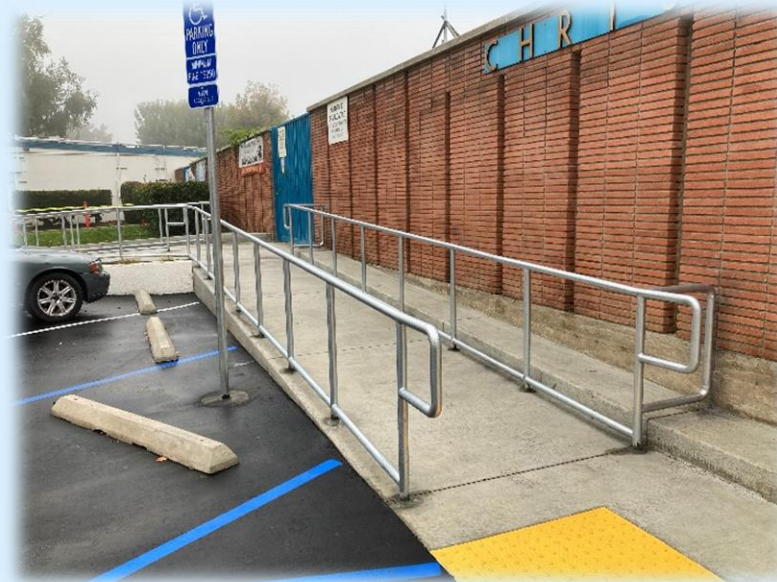
Accessible Parking and Ramp
