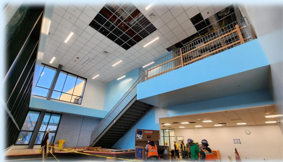
In Construction: Lobby
